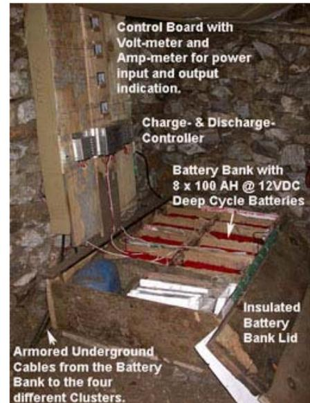
**Figure 3-4: Battery Bank well insulated in a locally made wooden box, designed to last 8-10 years, including the load growth.**
