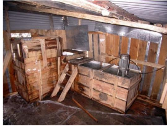
Figure 5: Inside the power house of the pico hydro power plant. The 1.1 kW generator is seen, with the wooden water canal, which cleans and streamlines the water for the propeller turbine's intake.
