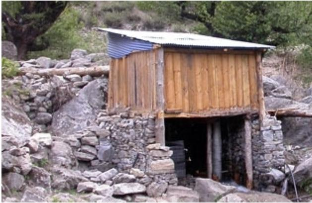
Figure 4: Beside the generator, the turbine and roof, the Pico hydro power plant infrastructure is built without any cement, using only locally available materials such as stone and wood, that creates a strong ownership among the users.
